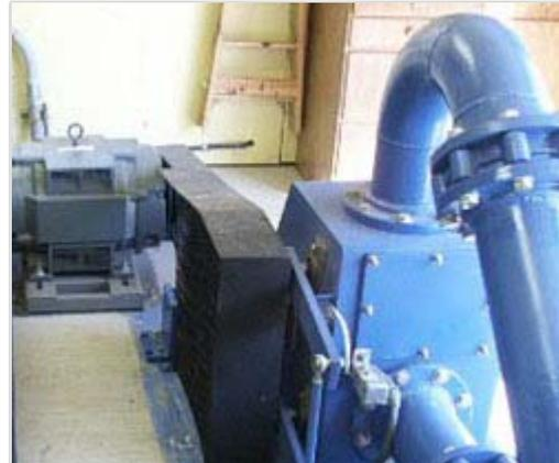
*Belt drive coupling between turbine and generator.*
